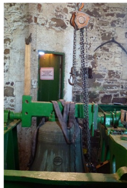
Bells lifted and bearings removed & cleaned Jan 24
