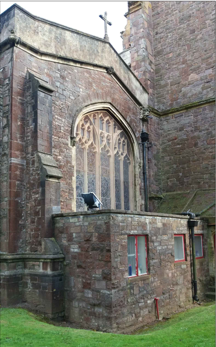
3. West End of North Aisle
