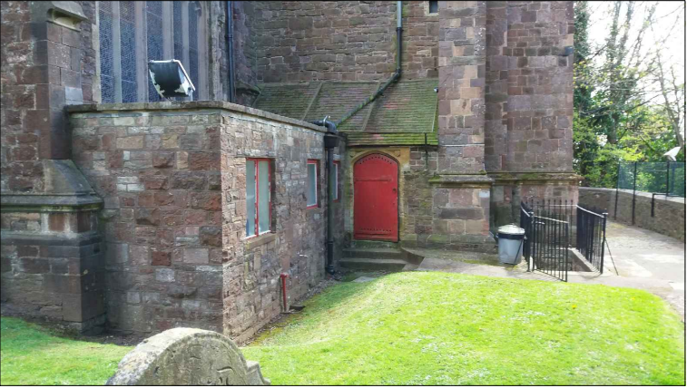
2. Existing toilet block and store room
